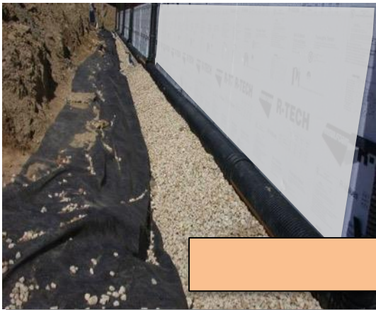
BELOW GRADE/SLAB INSULATION
