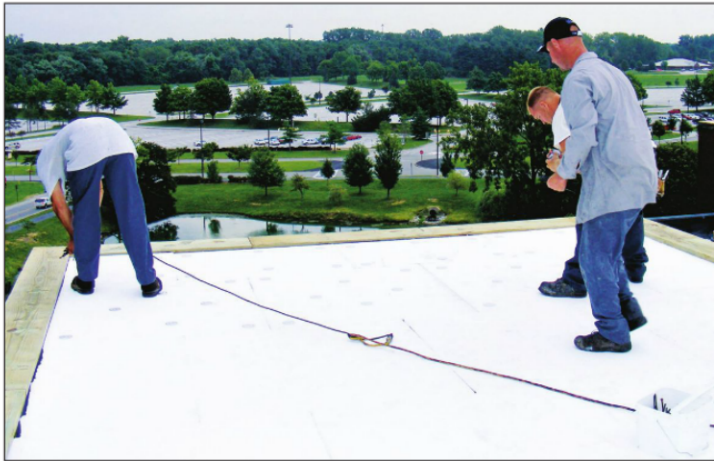
EPS insulation is light and easy to install, and costs significantly less in material and labour than other rigid foam insulations.
