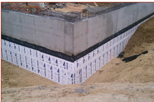
EPS insulation resists moisture better than XPS, including on buried foundations where it is in regular contact with wetted soil.
