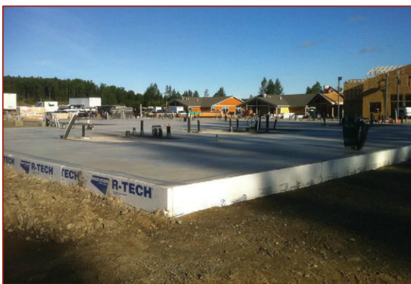
Rigid foam insulation is increasingly common in below-grade and under-slab applications.
