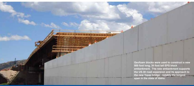
Idaho's heavily used trucking route and bridge (circa 1940) expands from 2 to 4 lanes to increase safety and capacity using InsulFoam<sup>®</sup> GF: Geofoam.
