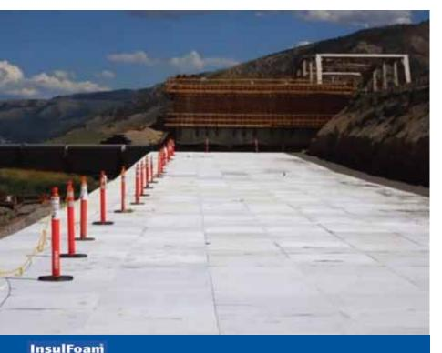
EPS block fill is partially installed, during bridge construction.
