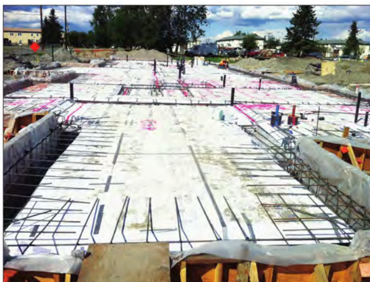
Rigid foam insulations, such as EPS, help insulate concrete slabs.
