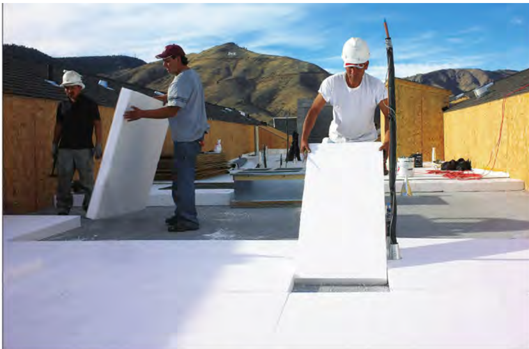
Contractors can readily cut EPS insulation to size in the field.
