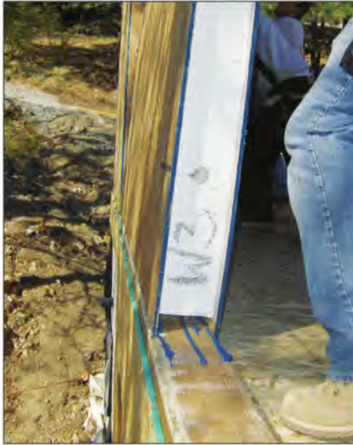
Structural insulated panels (SIPs) are typically made with an EPS core.
