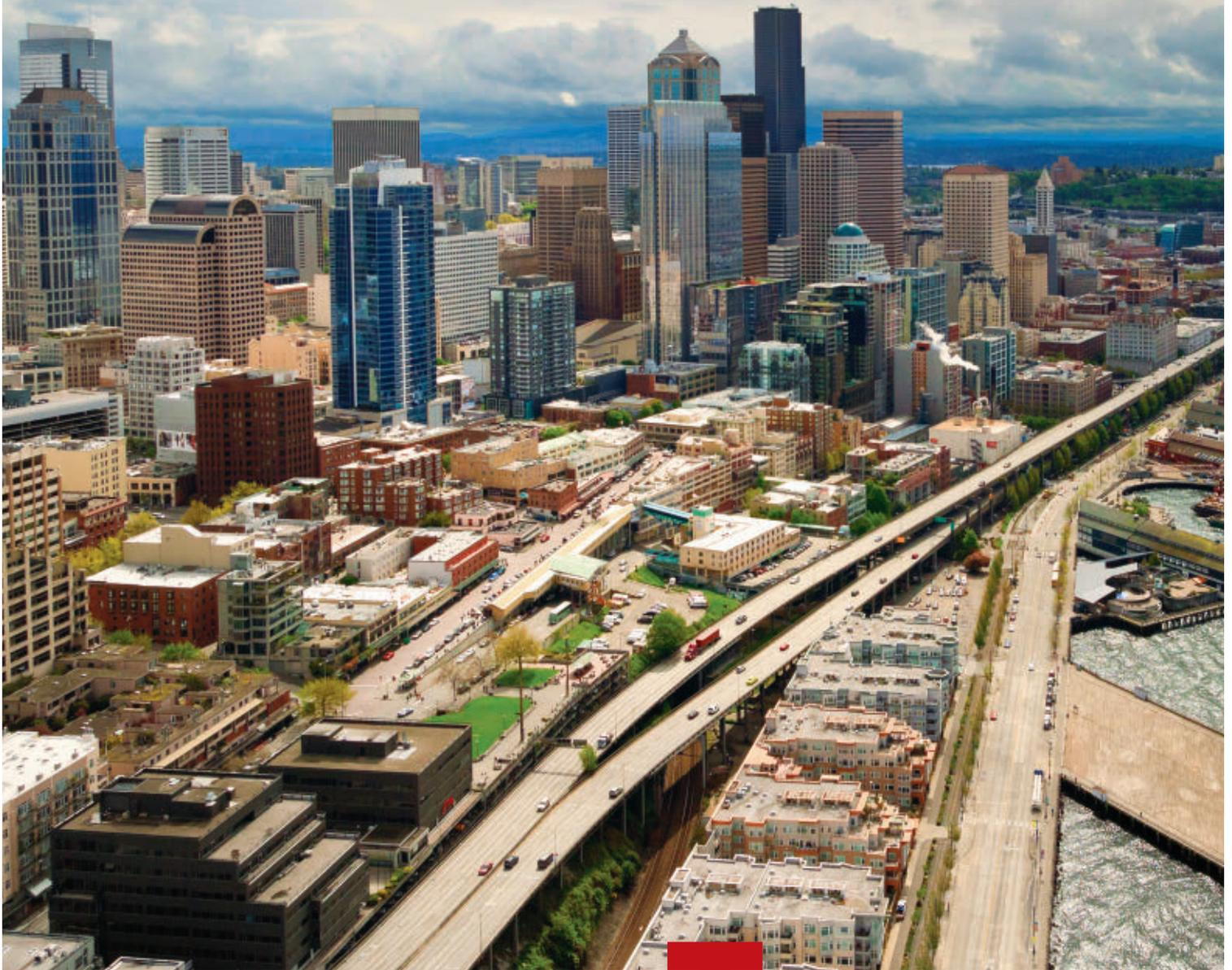
*The southern 1 mi stretch of Route 99 in Seattle has been rebuilt as two adjacent viaducts that cross active rail lines, roadways, and utilities. But what challenged the design team most wasn't the built environment but the extreme seismic vulnerability of the site.*
