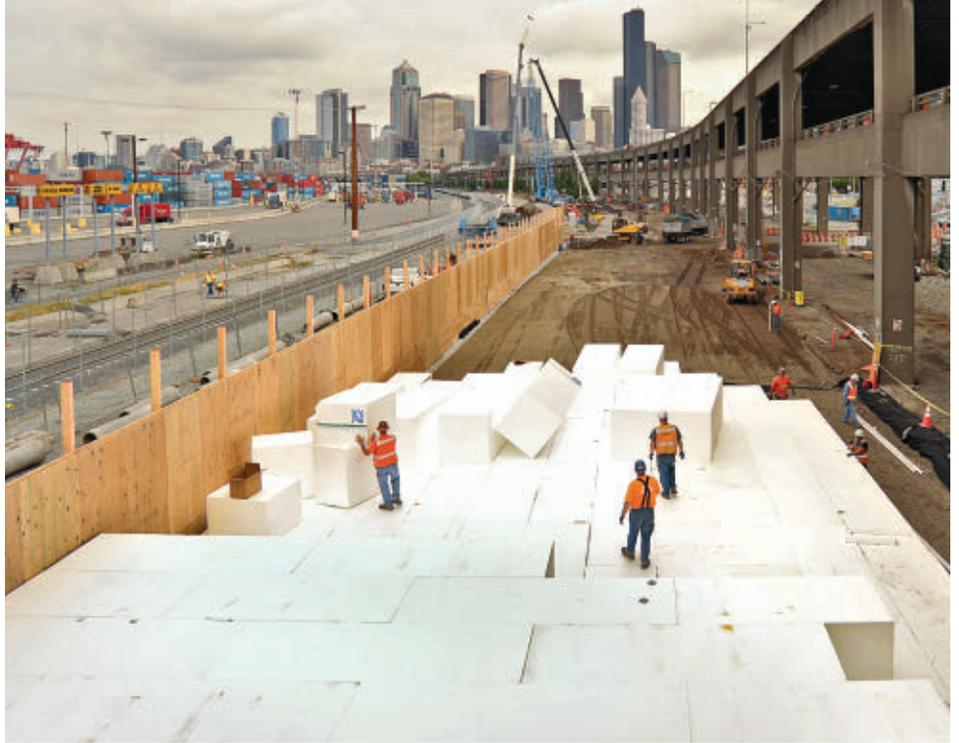
**Expanded polystyrene (EPS) geofoam was used as a lightweight fill. The EPS blocks can be easily cut and shaped to fit any embankment configuration and can be placed at rates of up to 1,000 cu yd per day, much faster than a gravel borrow embankment supported by a mechanically stabilized earth wall. After the EPS blocks are placed, they are covered with plastic to protect them from fuel or oil spills, and a roadway pavement section is then constructed over the EPS embankment.**
