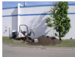
Excavation Site Minneapolis, MN Climate Zone 1
