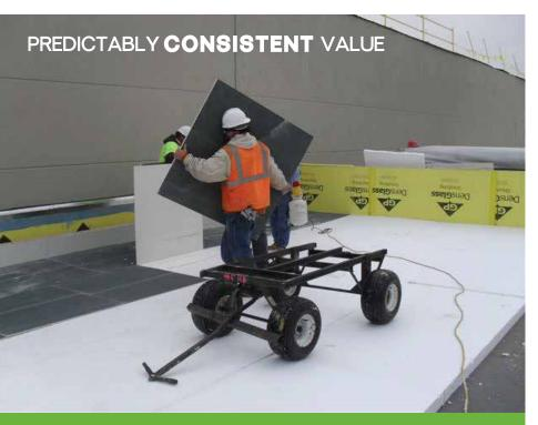
Insulfoam EPS tapered roof insulation offers the highest R-Value per dollar over other rigid insulations.
