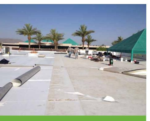
Insulfoam EPS tapered roof insulation offers the highest R-Value per dollar over any other rigid insulation.
