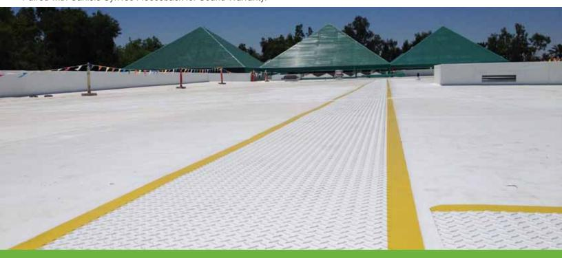
This Arizona tapered roof was installed with a single factory-tapered layer of 1.5 lb density InsulRoof Taper EPS insulation for long-term stable R-value, as well as added stability and
