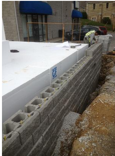
Even though it is very lightweight, geofoam is high-strength and suitable for a range of heavy loading conditions. Photo courtesy of Insulfoam
