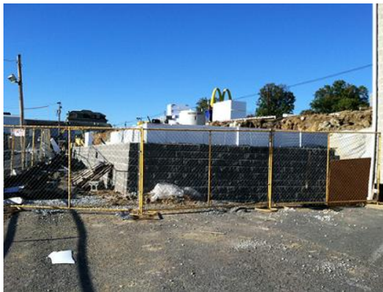
Projects built with geofoam include road beds, bridge approaches, levees and other jobs. Photo courtesy of Insulfoam
