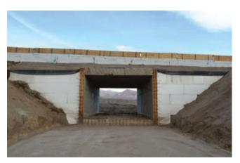
To avoid closing the highway, Granite Construction built a temporary wall for the culvert adjacent to the existing road, switched traffic onto two lanes built over it, and then excavated the existing highway to expand the culvert.
