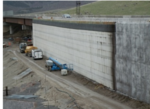
Shotcrete being applied on the vertical facia walls of the Topaz Bridge in McCammon, ID
