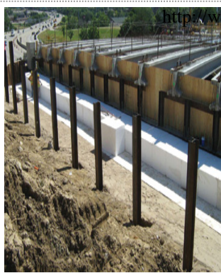
To widen the Pacific Street Bridge over I-680 in Omaha, Neb., Hawkins Construction excavated the soil between the existing abutment and soldier piles then formed and extended the abutment wall using EPS geofoam as lightweight backfill for the bridge approach.
