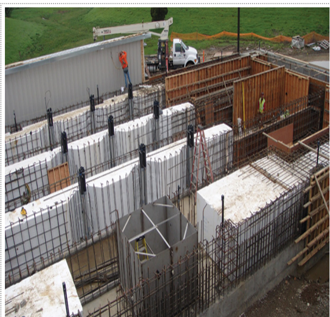
The contractor used EPS geofoam as a structural void fill in concrete forming operations for water channel walls in the Fairfield-Suisun Sewer District, Calif., water treatment plant.
