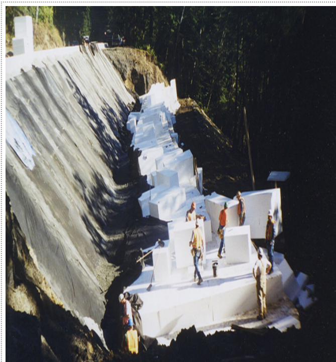
EPS geofam's low weight makes it an excellent option for stabilizing steep slopes without the need to change the final slope geometry.
