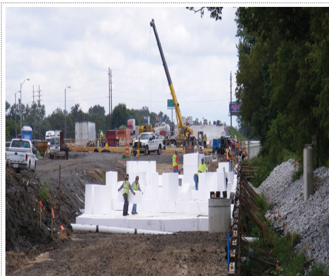
To enable a shallow over-excavation of high-organic-content soils, Walsh Construction used EPS geofoam blocks as fill to widen the I-80/I-65 interchange in Gary, Ind.
