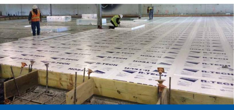
By utilizing EPS instead of XPS, the concrete contractor saved approximately \$20,000 in material costs.
