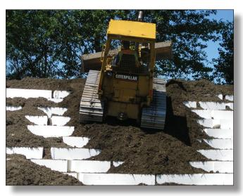
unaffected by freeze-thaw cycling, moisture, and road salts. Other fill materials such as wood chips, saw dust, lightweight concrete and soil can be weather sensitive during installation.
